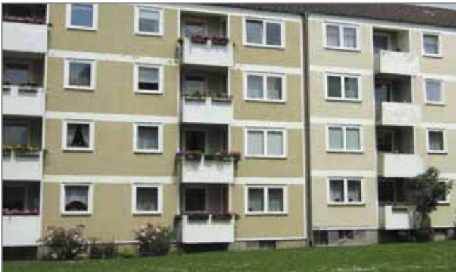
The large housing estates of the 1950s to 1970s often need modernization
